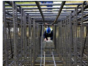
Diaphragm Wall Reinforcement
