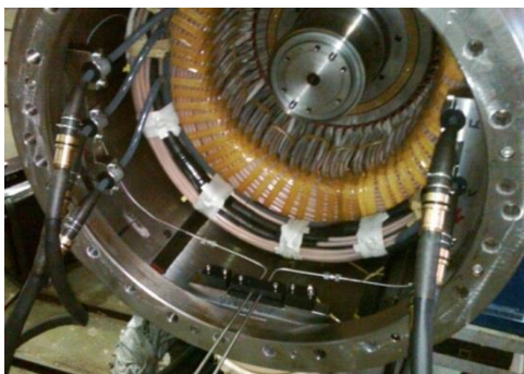
Motor winding temperature
