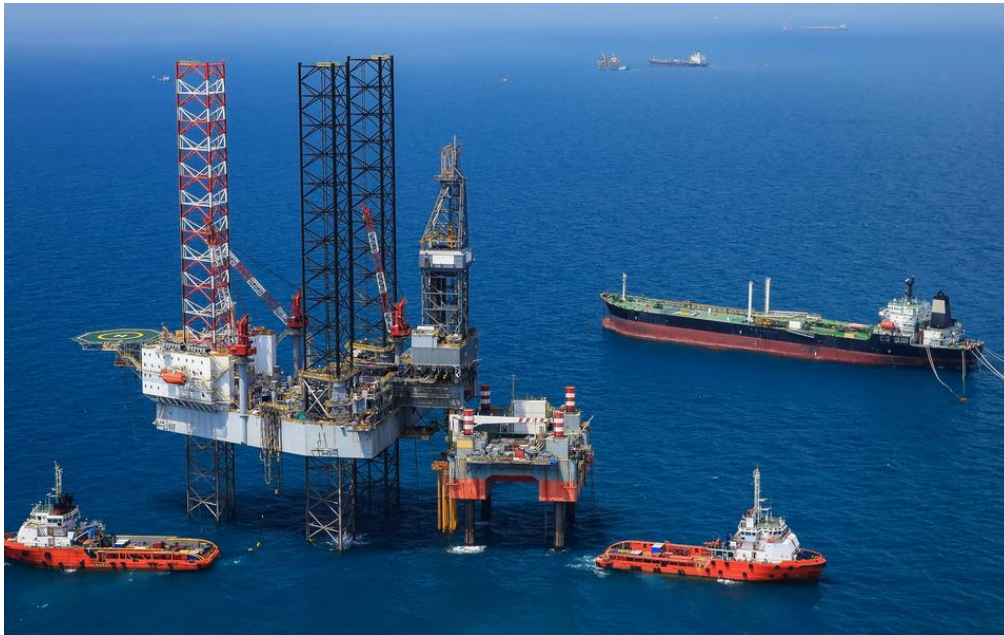
Figure 3. A jacking rig with three “legs” in the application for oil production in the sea. In total 18 or 24 motors per pillar are used for driving [2].
