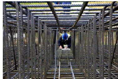
Diaphragm Wall Reinforcement
