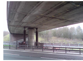
Motorway Bridge Deck and Soffit
