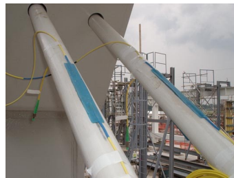
Airport Roof Structure
