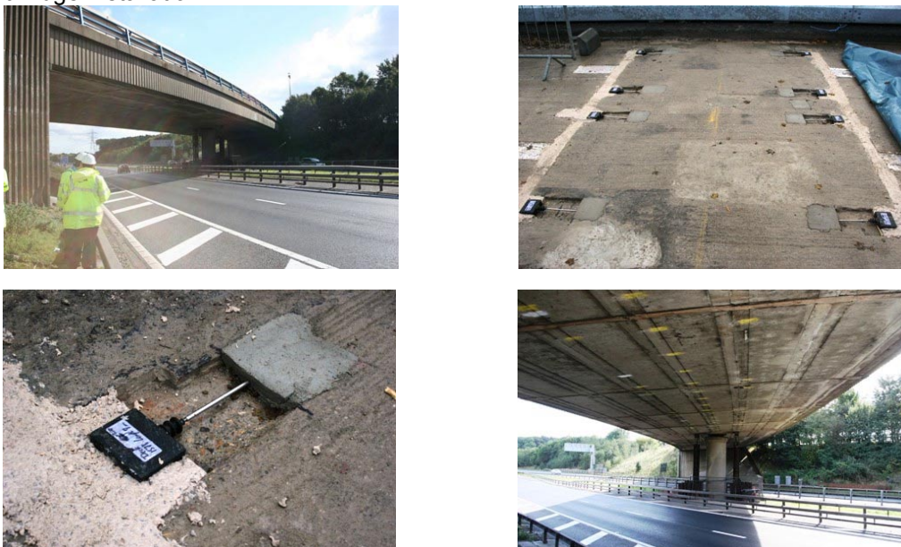
Motorway Bridge Deck and Soffit
