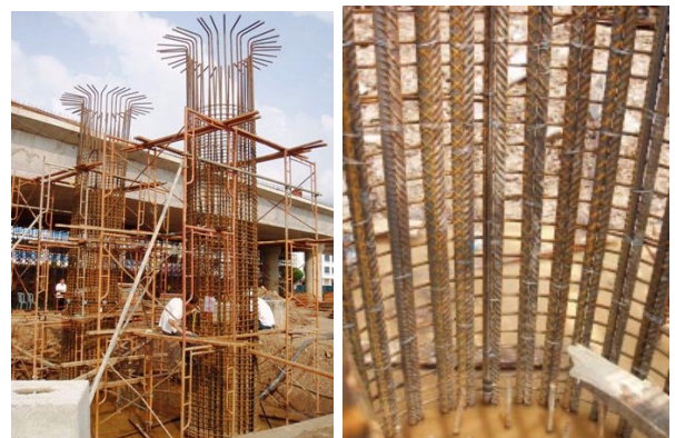
Road Bridge Pier monitoring, Malaysia
