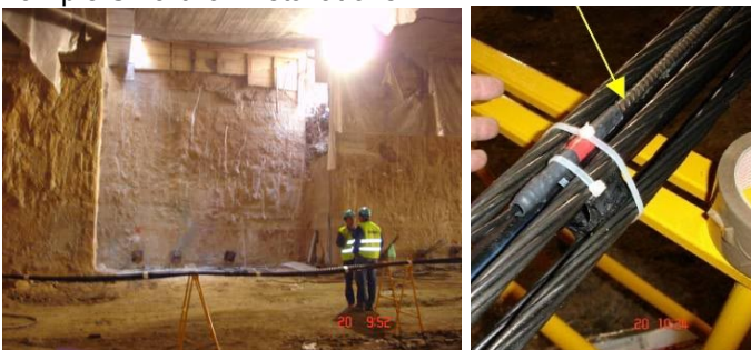
Diaphragm wall ground anchor tension, Spain
